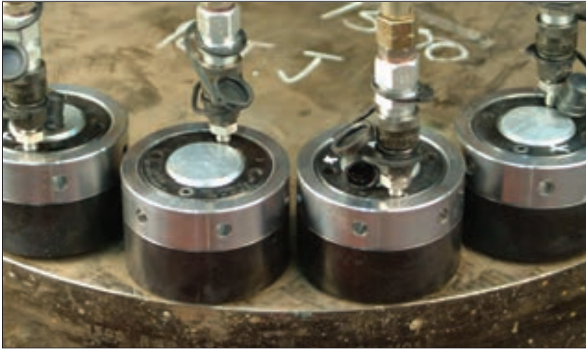
▲ Tensioning with hydraulic nuts.
