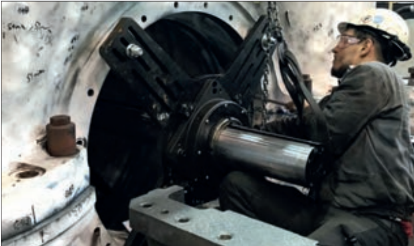
▲ Pipe cutters and weld preparation.
