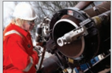
▲ Pipe cutters and weld preparation.
